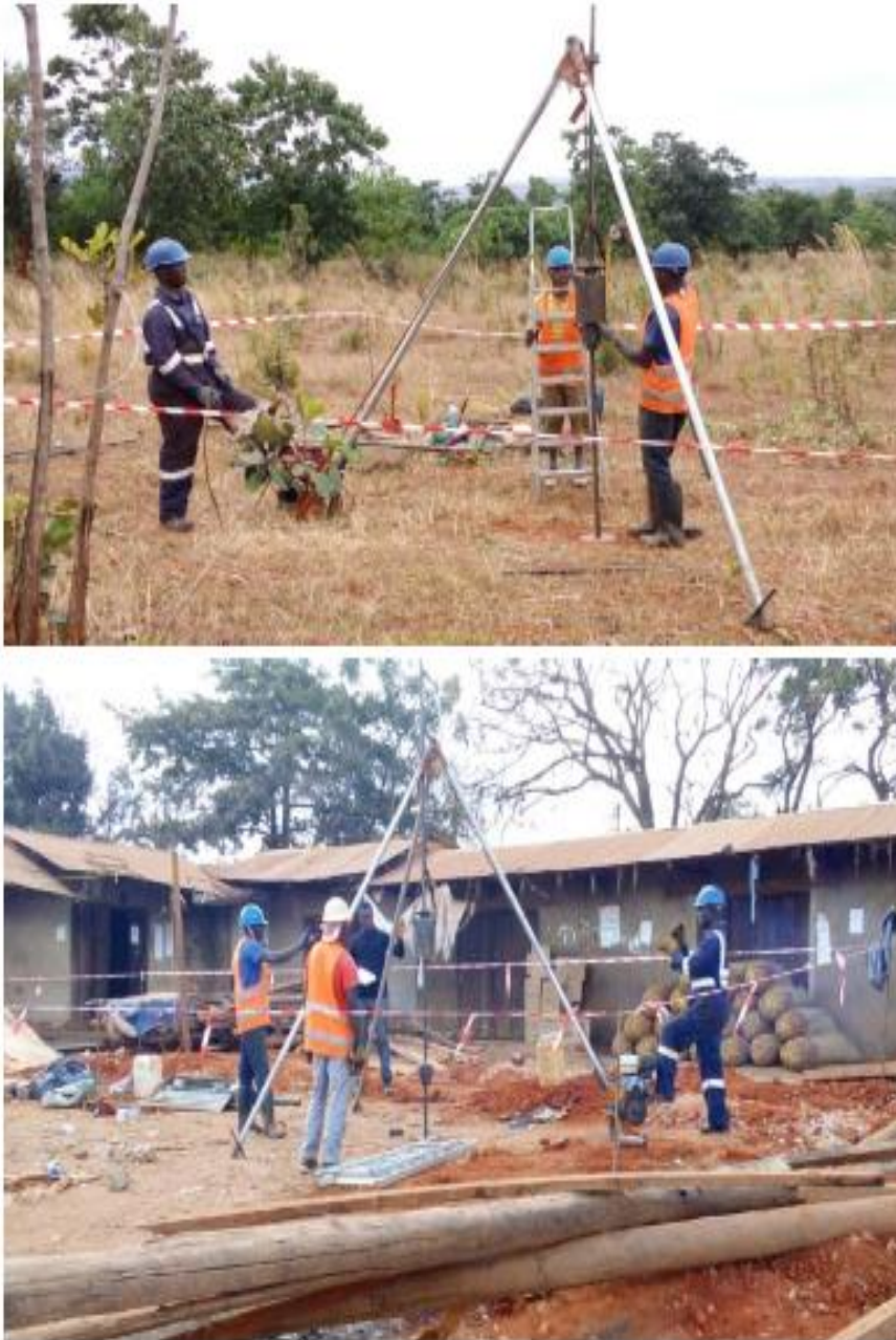
Figure 5-2 –Selected DPSH photo at Lilambo Industrial Area and Manzese A market
