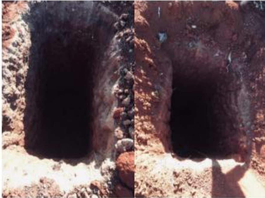
Figure 5-1(a) –Selected trial Pit (TP01 & TP02) photos at Manzese A Market
